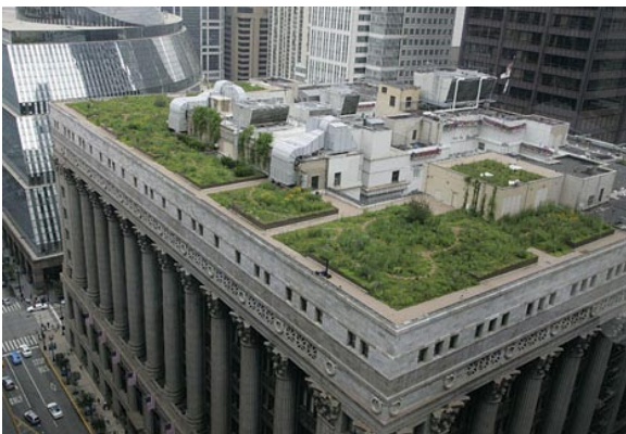
Green Roof, McDonough + Partners, Chicago
